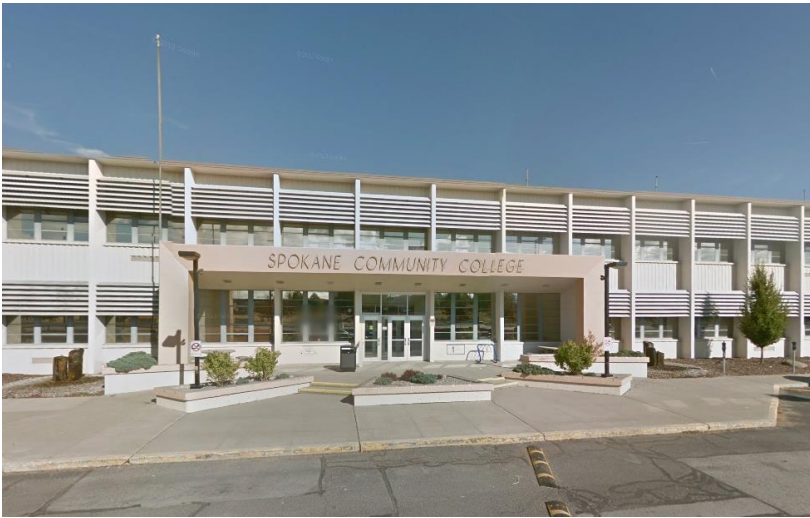
Main Entrance From the South Side (along Mission Ave.)
