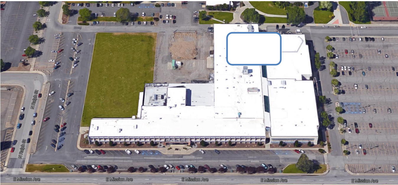
Building 01 (Old Main) in the Southwest Corner of Campus (Intersection of Mission and Greene) (Blue Rectangle locates the CAD & Mechanical Program area) (Visitor Parking and Parking Meters available along the front of the building)
